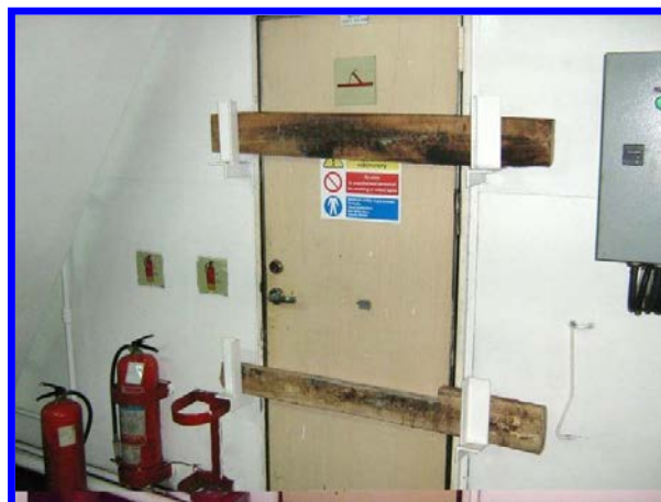
As above – a further deterrent to access should the lock be breached (metal is preferred to wood)
