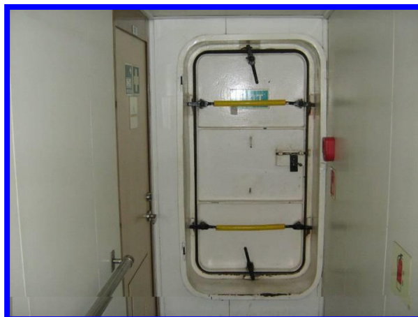
Watertight door effectively secured
